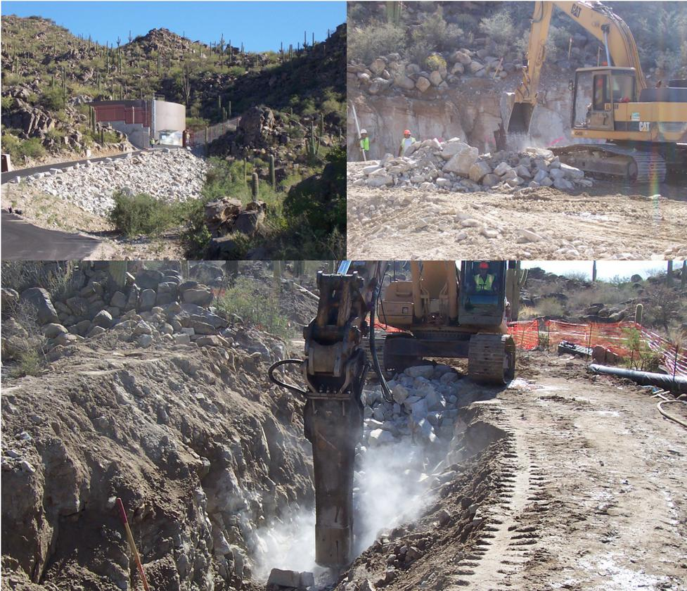
Construction of a new 1800 ft. water plant access road, site work including the installation of approximately 300 lineal feet of concrete retaining wall, and the installation of a 500,000 gallon welded steel potable water reservoir.
