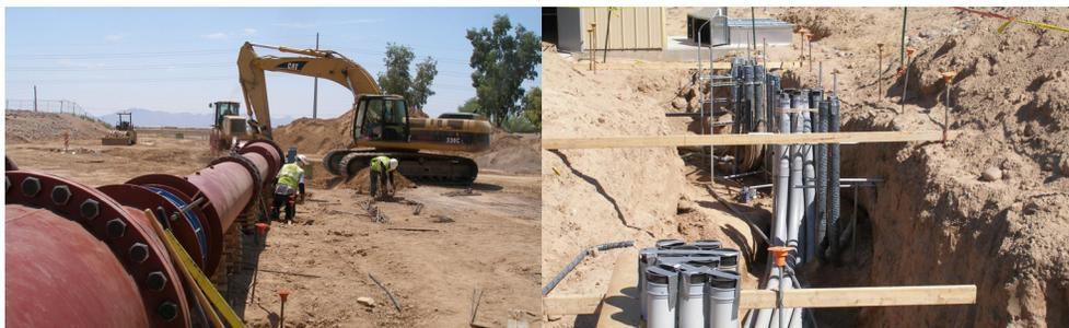
Construction of a new recharge facility pump station, modifications to an existing wet well structure and upsizing the existing aquifer storage and recovery (ASR) wells.
